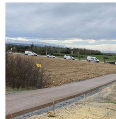
Béton poreux Castres (81) Source: Agilis
