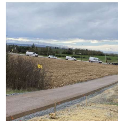
Béton poreux Castres (81) Source: Agilis
