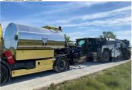
UN MALAXAGE ET LES DERNIERS AJUSTEMENTS EN TENEUR EN EAU JUSQU'A L'OBTEMTION DE LA TENEUR OPTIMALE SE FONT EN INJECTION D'EAU DIRECTEMENT DANS LA CLOCHE DU PULVIMIXEUR (O JACOB GOUVENAUX BRIJA VESSIONE).
