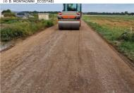
LE COMPACTAGE DU MATERIAU TRAITE A L'AIDE D'UN COMPACTEUR MONOBIL LISSE VIBRANT, (© B. MONTAGNINI ECOSTAB)
