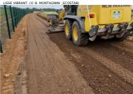
REGLAGE FIN DE LA PLATE-FORME TRAITEE A L'AIDE D'UNE NIVELEUSE. (© B. MONTAGNINI \_ECOSTAB)
