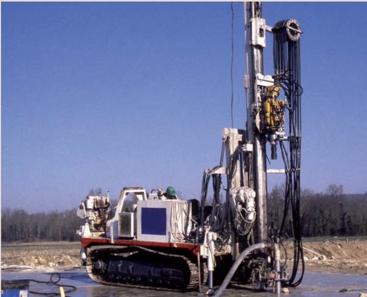
→ Atelier de forage de jet grouting.
